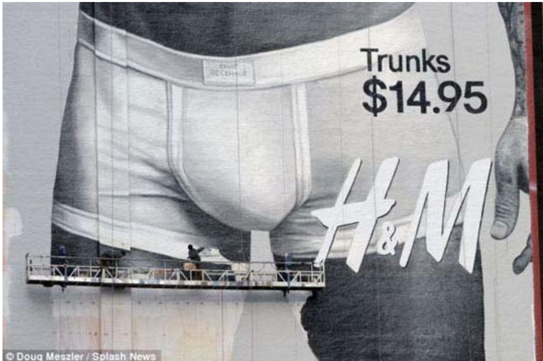
Sign Installation, NY Times Square
